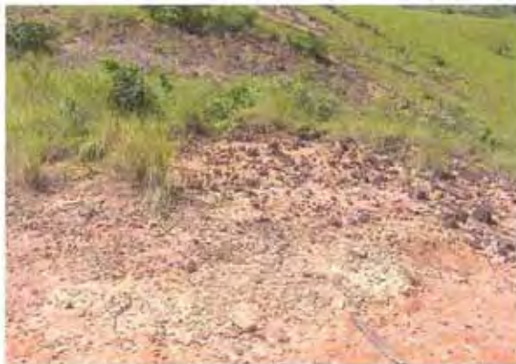
Soil erosion at ridge
