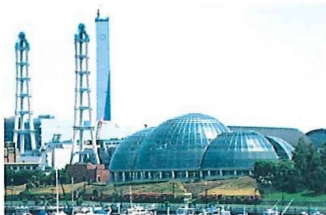
Application of heat from garbage incinerators (Tropical Greenhouse Dome, Tokyo)
