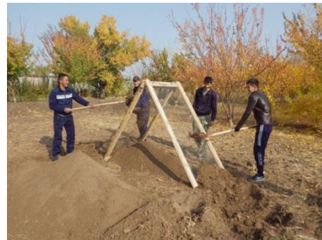
Photo 6 Soil sieving work
